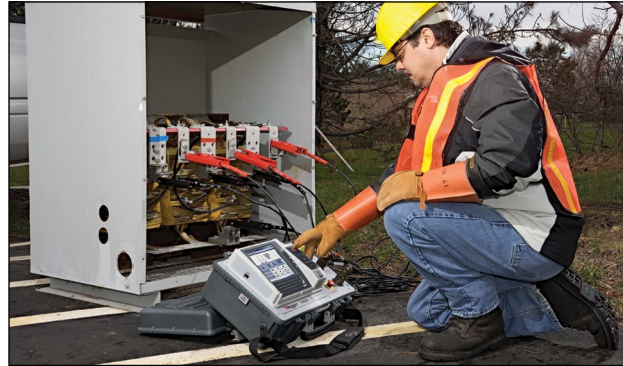
TTR330 shown testing a pad mount three-phase transformer
